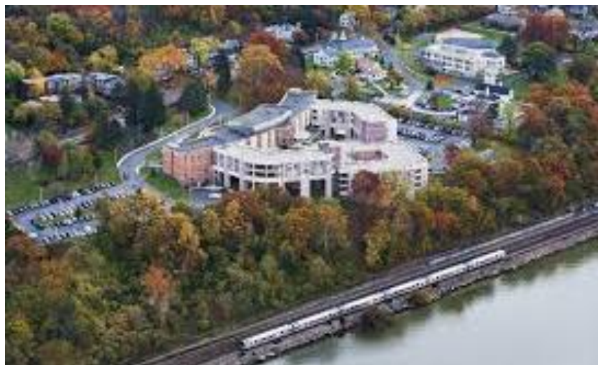
An aerial view of Cabrini of Westchester along the Hudson River in Dobbs Ferry, NY.
